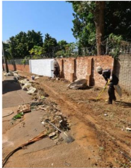
Progress made on cleaning up the corner.
